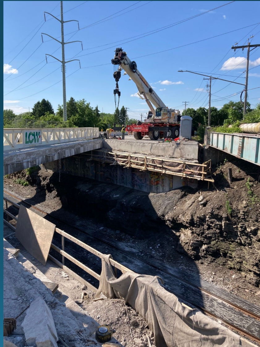
E Brighton Ave over railroad, Syracuse. Source: Syracuse
