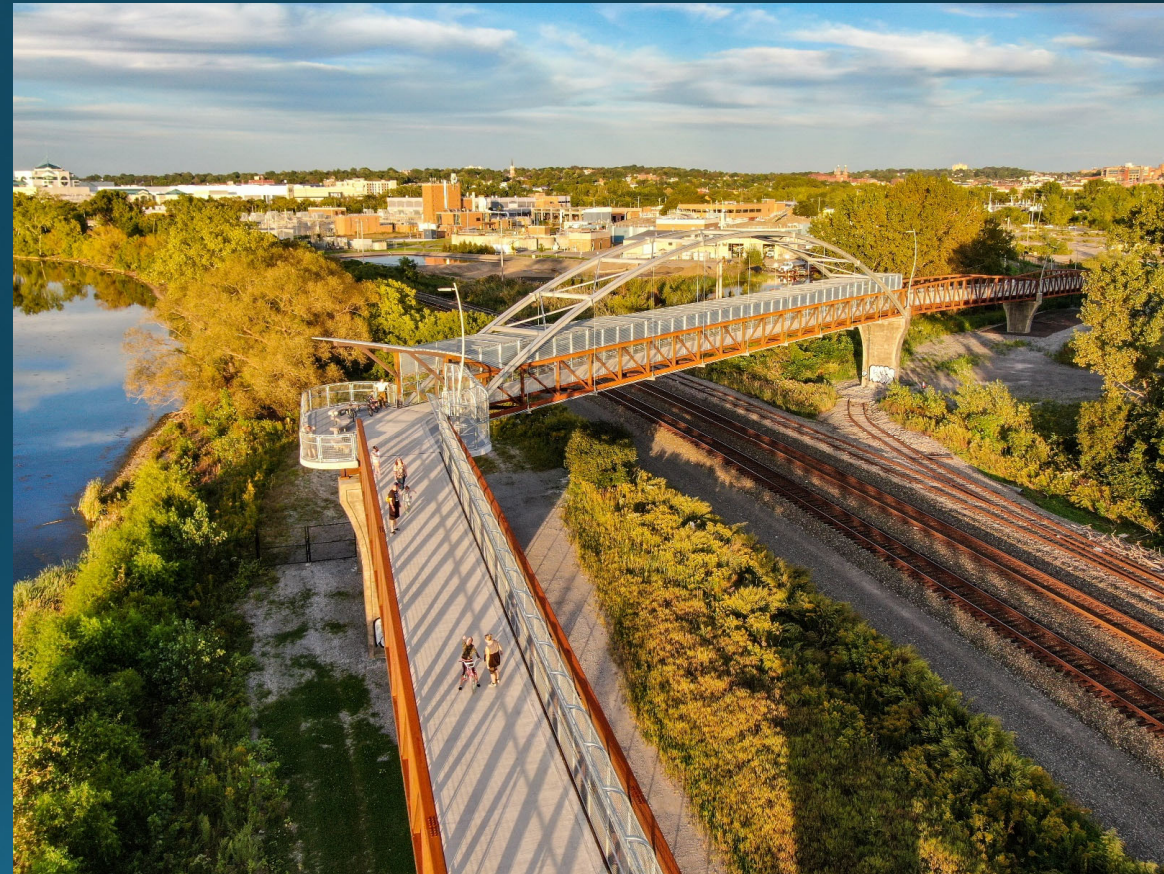
Onondaga County Loop the Lake trail bridge over CSX. Source: Onondaga County
