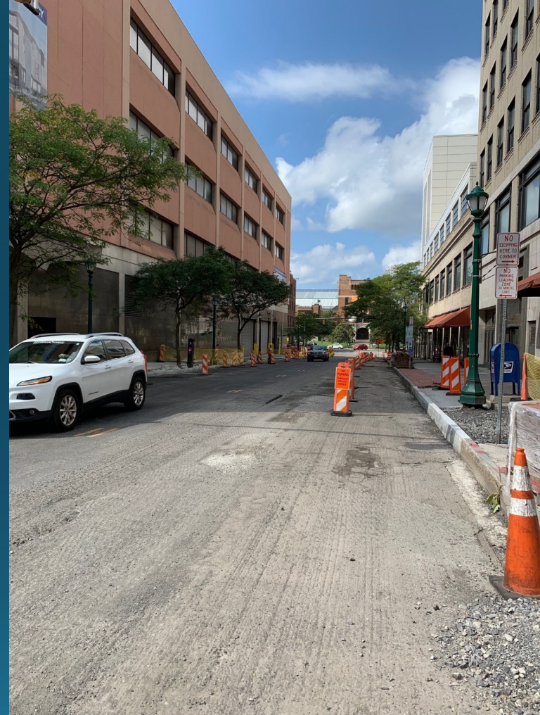
E Jefferson St paving, Syracuse.
