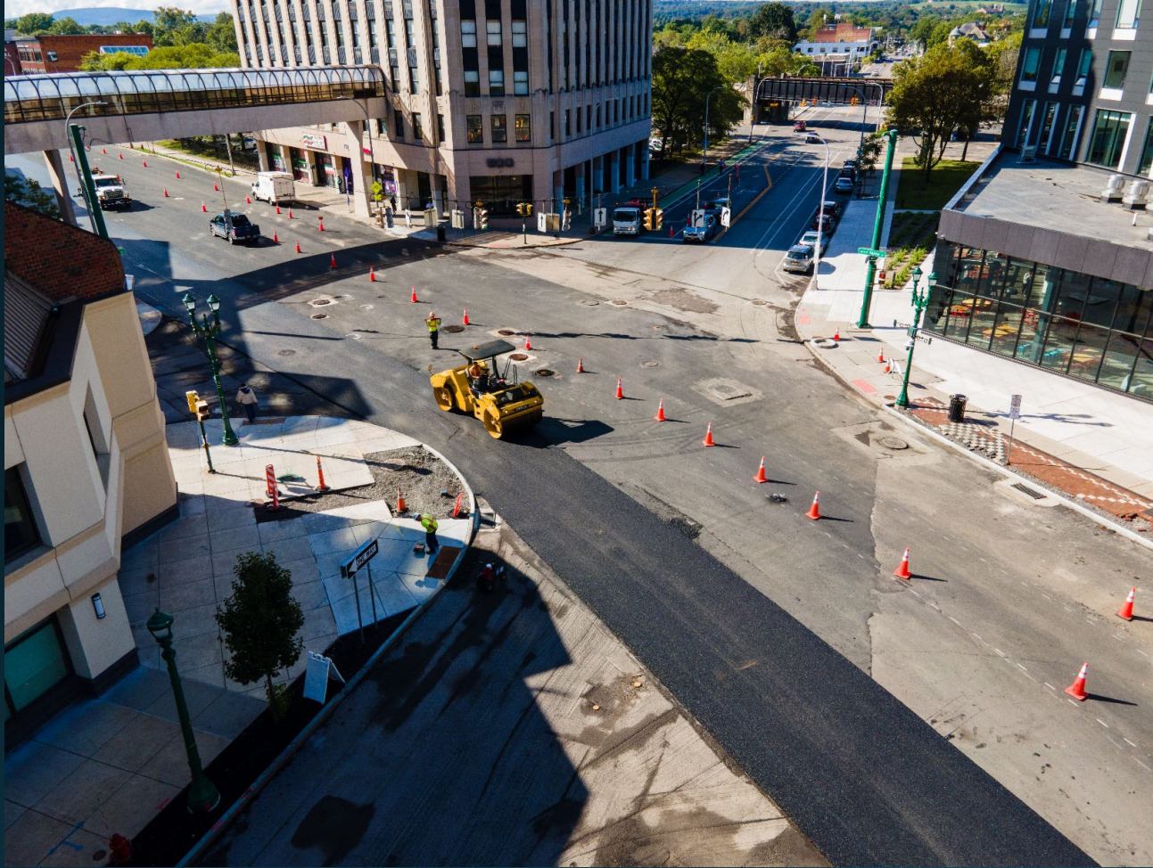
S Salina St paving by Harrison St, Syracuse. Source: Syracuse
