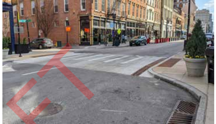
Raised crosswalk in Cincinnati, OH
