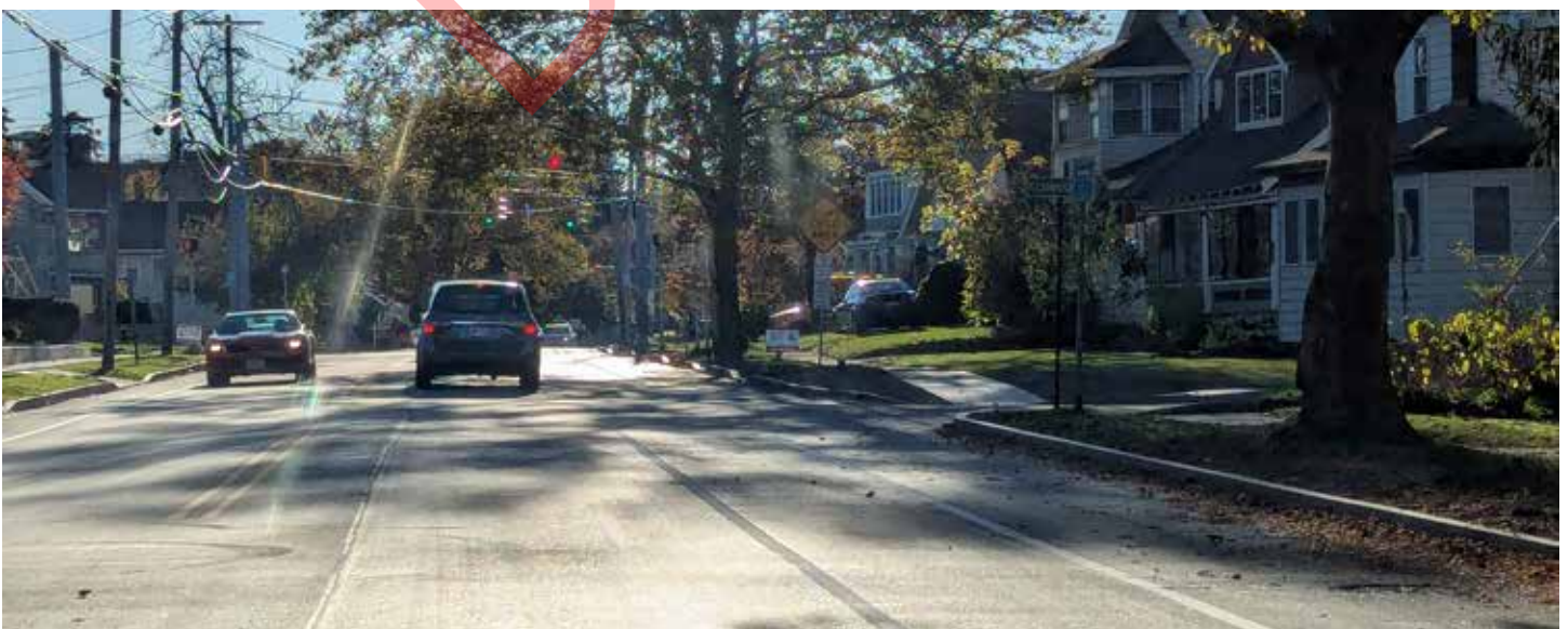
From Top: Looking north on N Midler Ave towards the Town of DeWitt; Complete streets treatments in Downtown Syracuse; Looking west on Court St near 7th North St.
