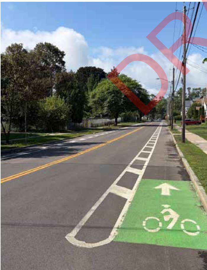
Buffered bike lane along Court St in Syracuse.
