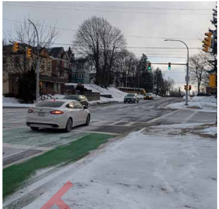
Bike and pedestrian infrastructure at the Grant Blvd / Court St intersection.
