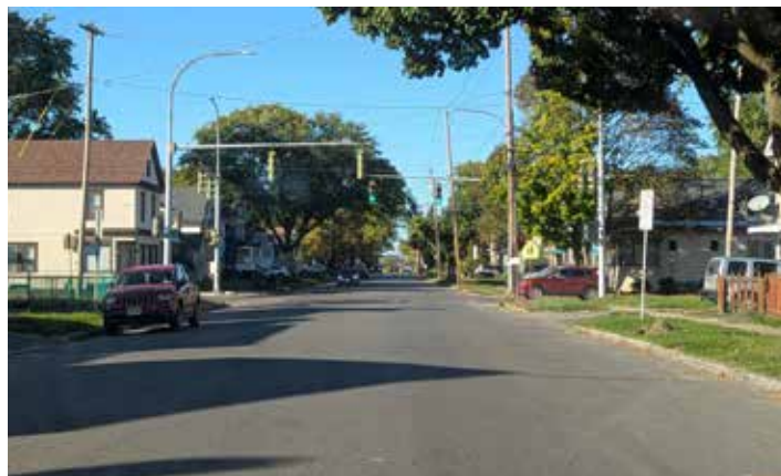
N Midler Ave / Tyson Pl intersection, looking north.
