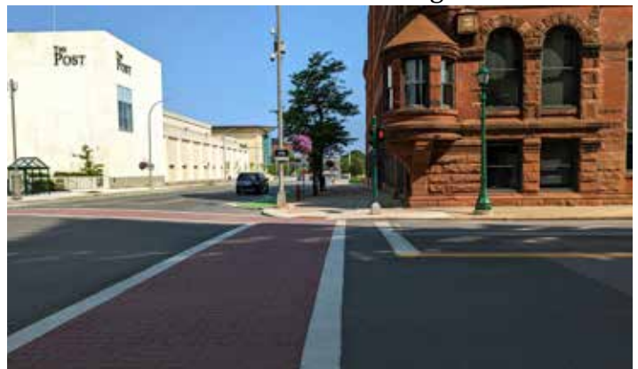
Enhanced crosswalk in Downtown Syracuse that mimics a brick pattern to stand out from the pavement.
