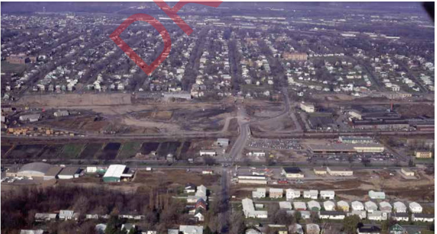
Looking north along Midler Ave during the construction of I-690 in the 1960s.
