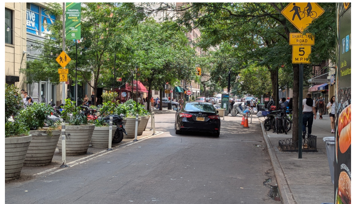
Chicane, utilizing planters and flex posts, in New York City
