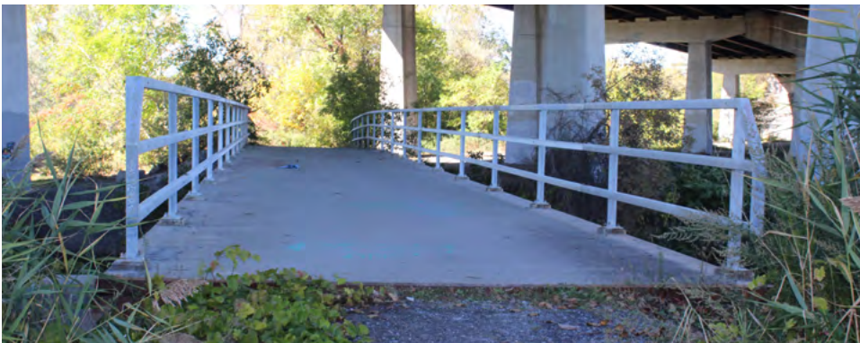
Image 7: Bike/pedestrian bridge over Ley Creek along Ley Creek Trail under I-81 overpass
