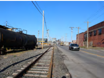
Image 25: Active rail spur along Hiawatha Boulevard
