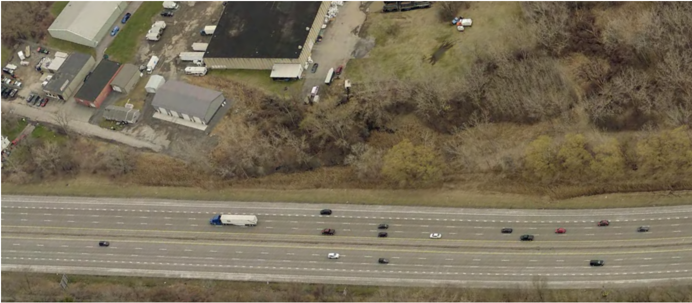
Image 49: End of Luther Avenue connecting to I-81 right-of-way Source: Eagleview, 2024
