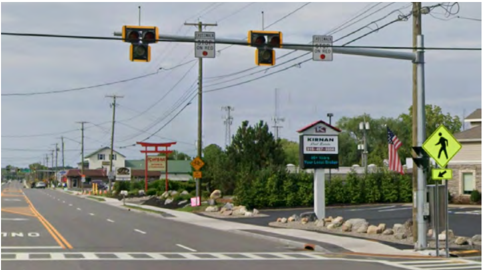
Image 44: HAWK signal on Old Liverpool Road Source: Google Street View Sep 2025
