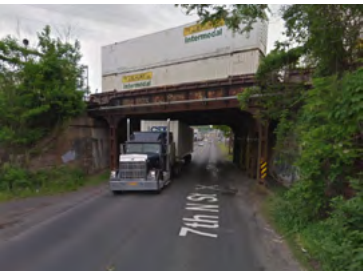
Image 24: CSX rail bridge over 7th North Street Source: Google Streetview
