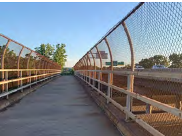
IMAGE 4: Bear Trap Creek Bikeway bridge over I-90
