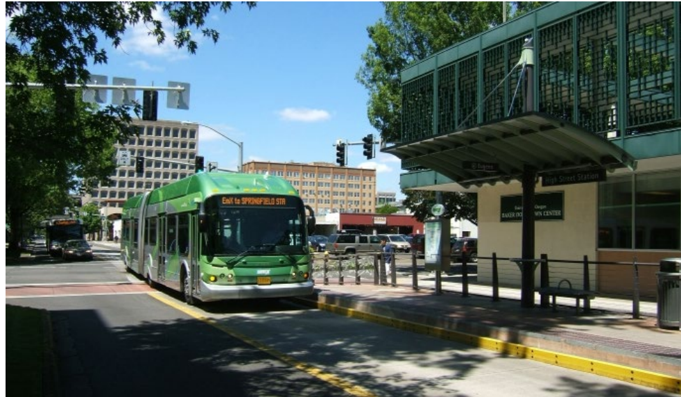
Figure 5: An EmX station with level boarding. (Image Source: Transportation for America)
