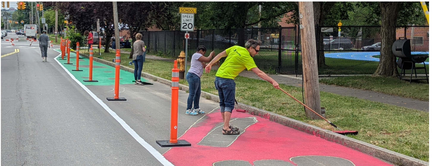
Volunteers work on a painted chicane behind STEAM at Dr. King Elementary as part of the Reconnecting Communities planning grant.
