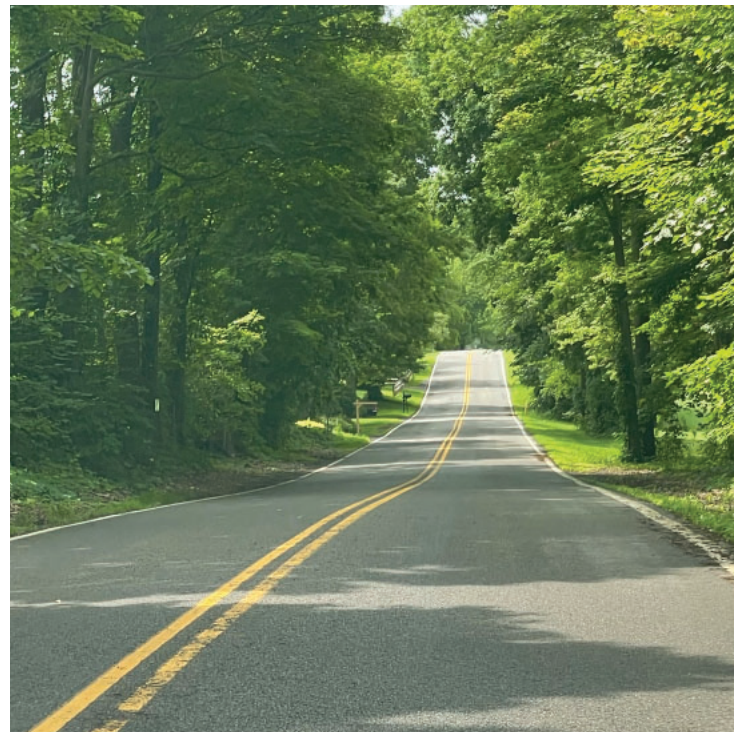
Figure 3b. Duguid Road has a limited shoulder that could be widened to provide safer conditions for both cyclist and pedestrians.
