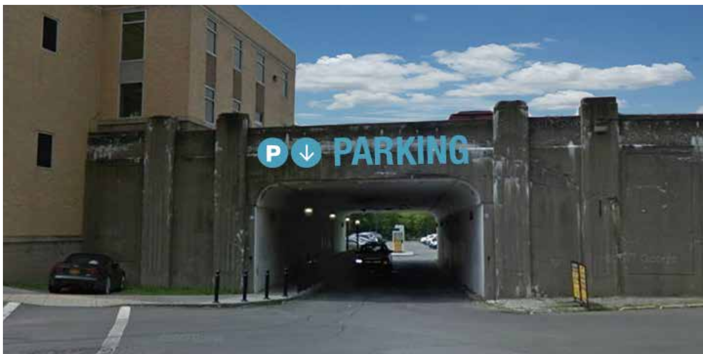
Recommended signage for the Trolley Lot in Armory Square from the Armory Square Mobility Study.
