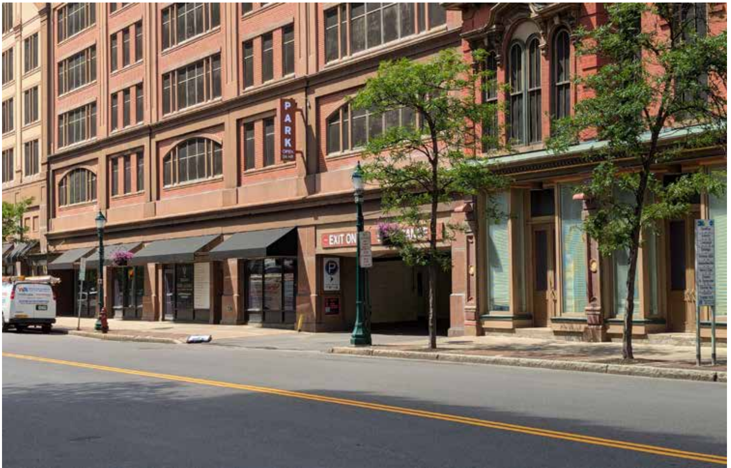
The Treasury Parking Garage is partially located within the former Larned Building. After a fire severely damaged the interior of the building, the structure was converted into a garage while preserving its facade.
