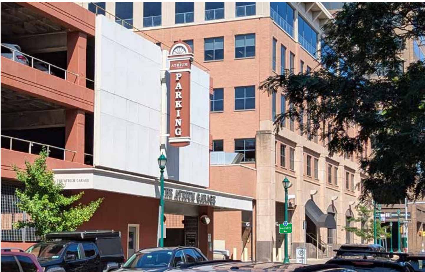
24x16 sign by the Atrium Garage.
