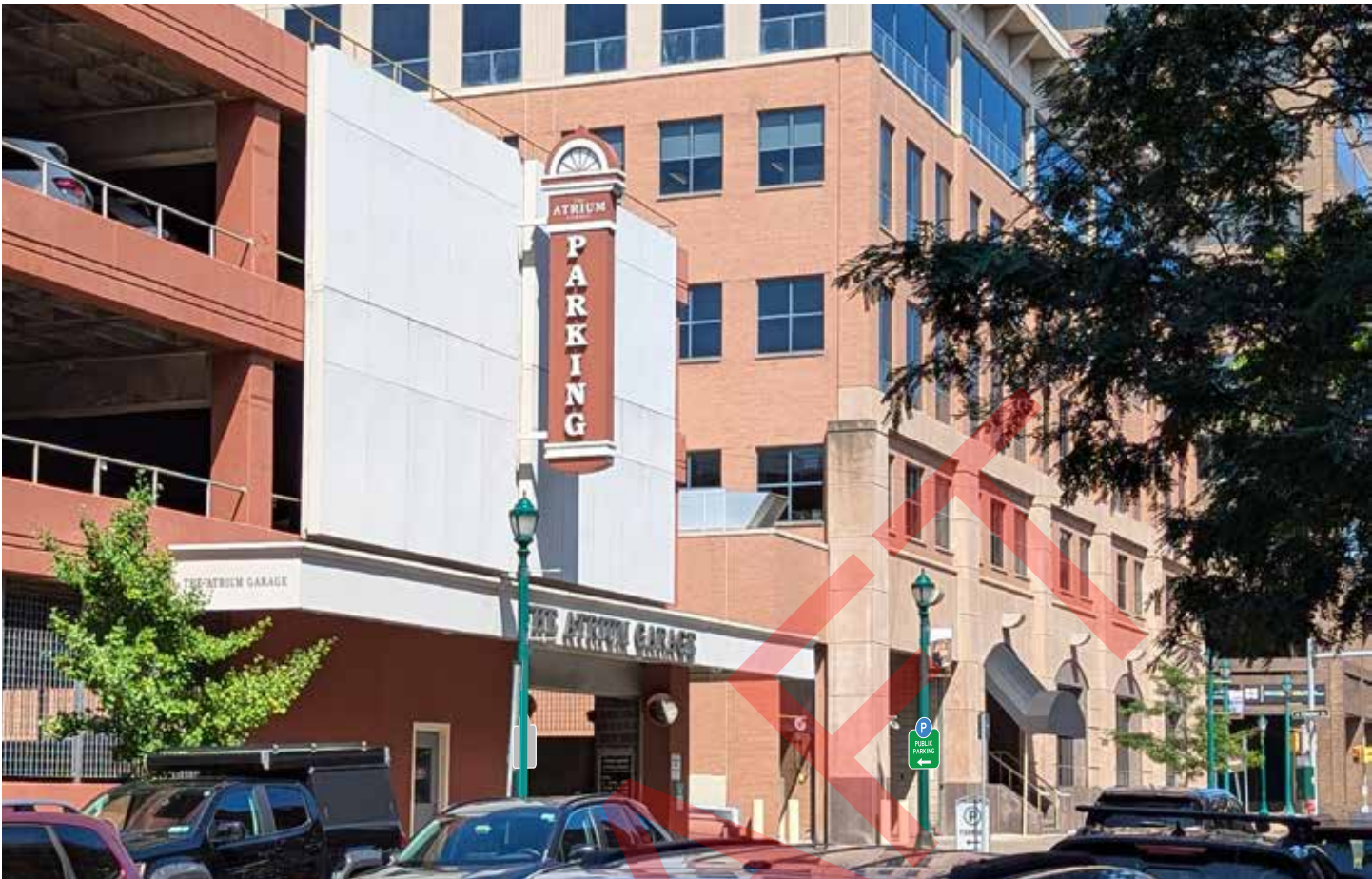
16x16 sign by the Atrium Garage.
