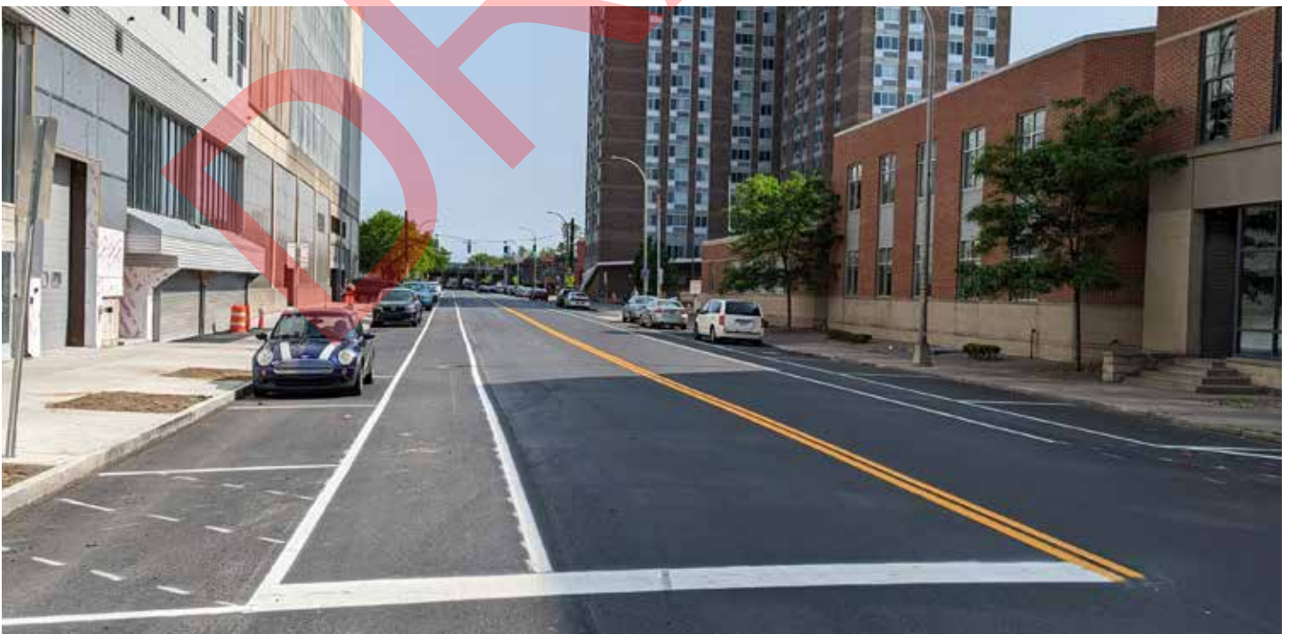
S Clinton St, from W Jefferson St to W Taylor St, has been converted to two-way traffic, as recommended within this study.
