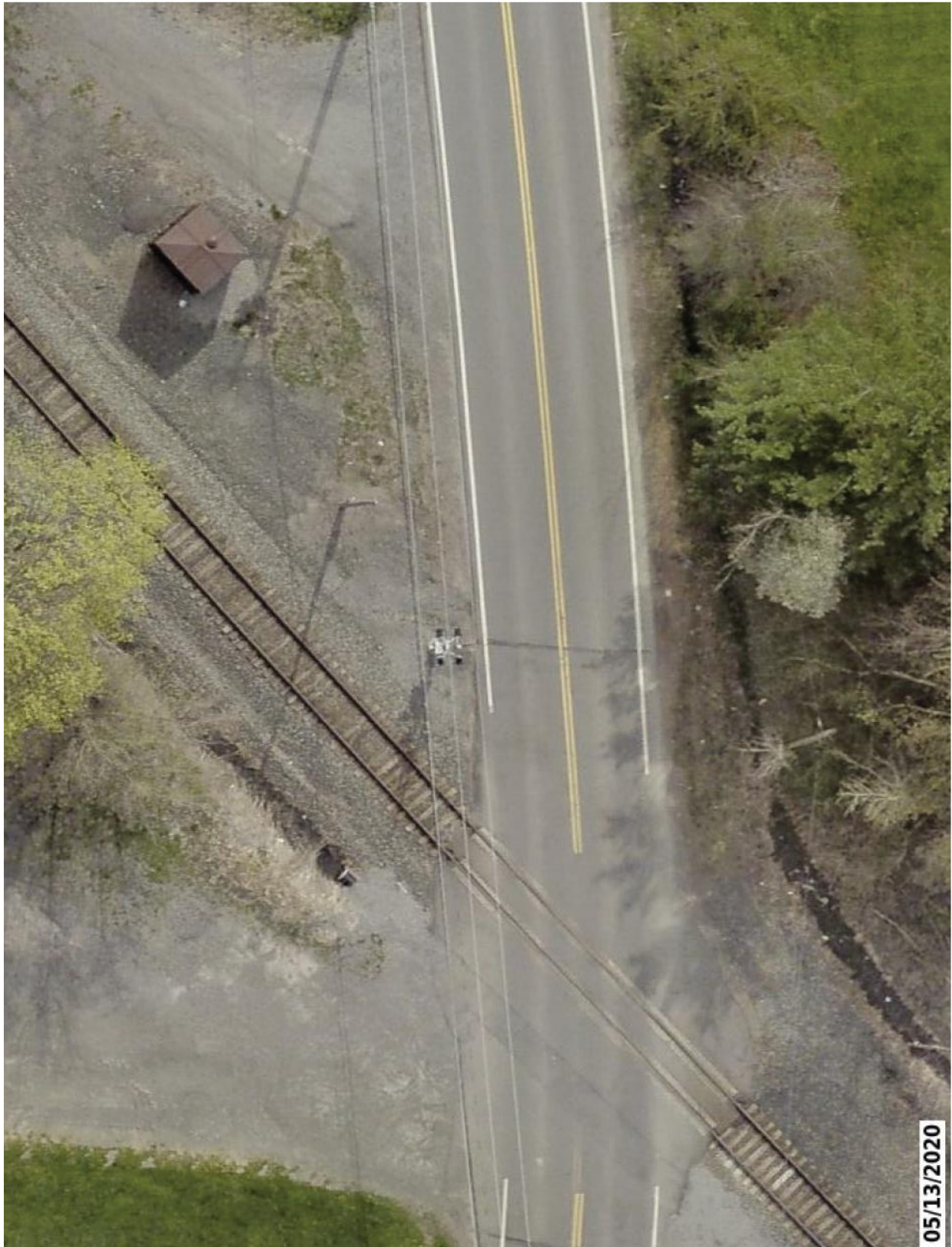
Figure 12 – Existing Conditions: CSX Railroad crossing at Guy Young Road
