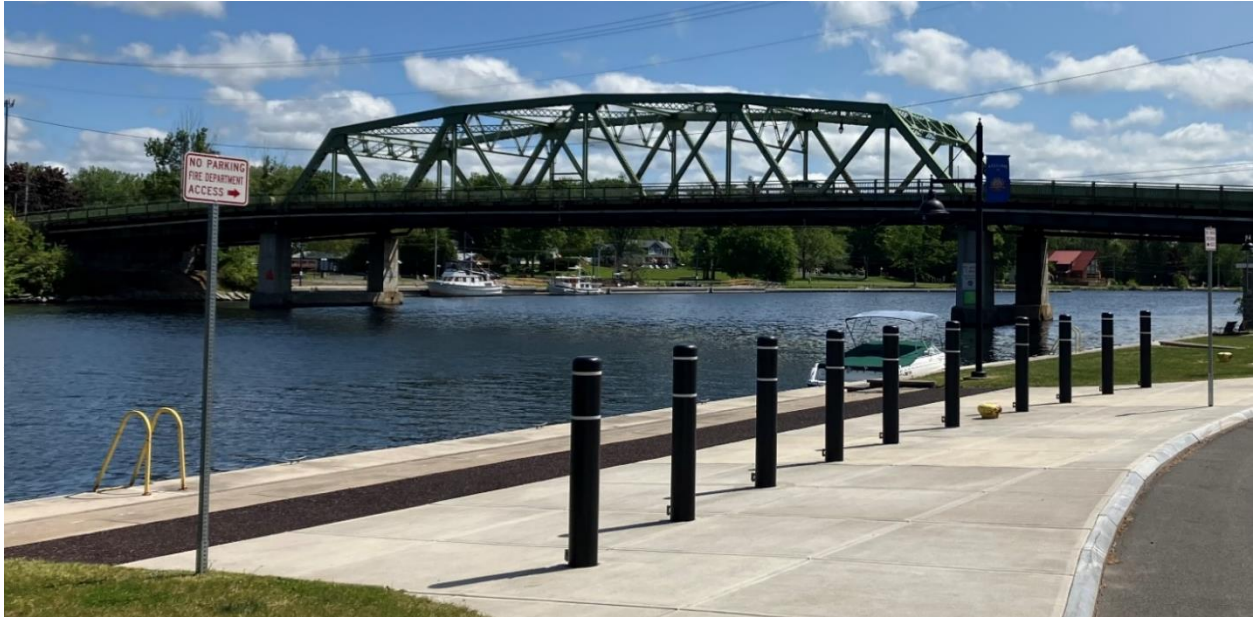
Figure 13 – Brewerton Route 11 Truss Bridge over Oneida River (looking east)
