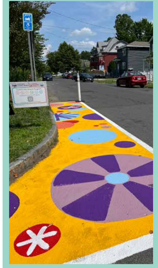
Temporary flex posts are used at the corners of the painted curb extensions to reinforce the visual narrowing of the roadway.
