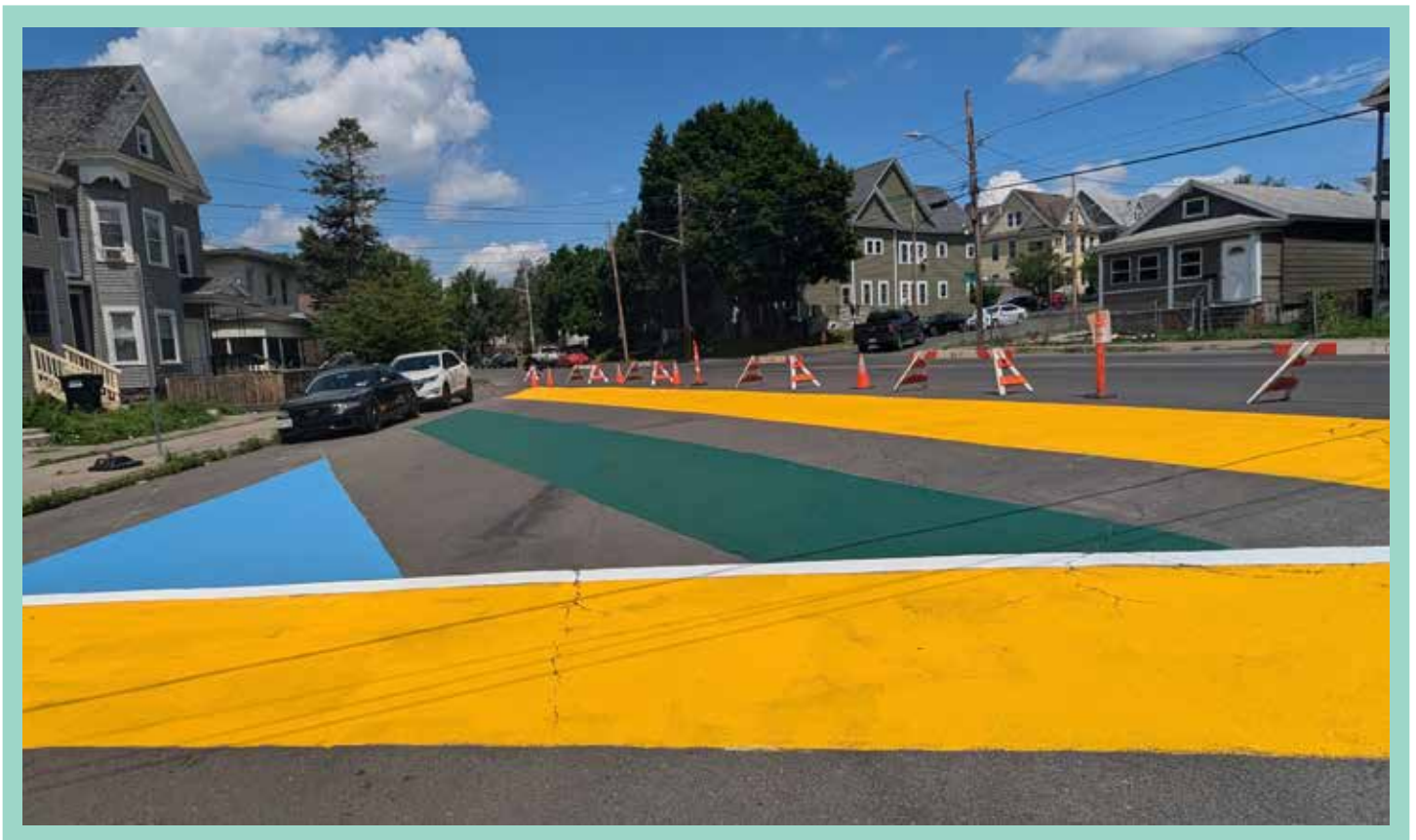
Large painted stripes were intended as a transition zone between vehicle traffic and the temporary pedestrian plaza on the Northside.
