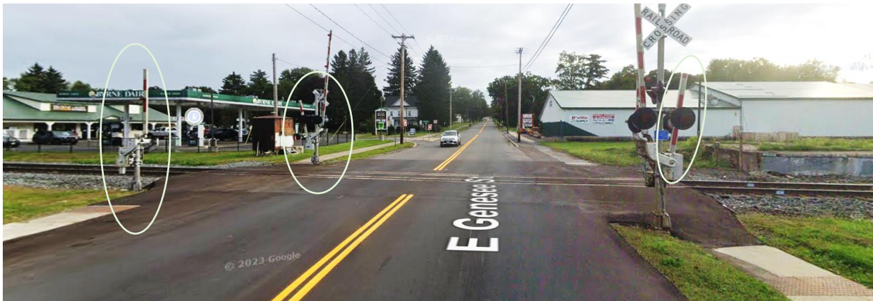
Figure 14 – Example of pedestrian crossing gate, Route 31 (E. Genesee St.) Baldwinsville, NY.
