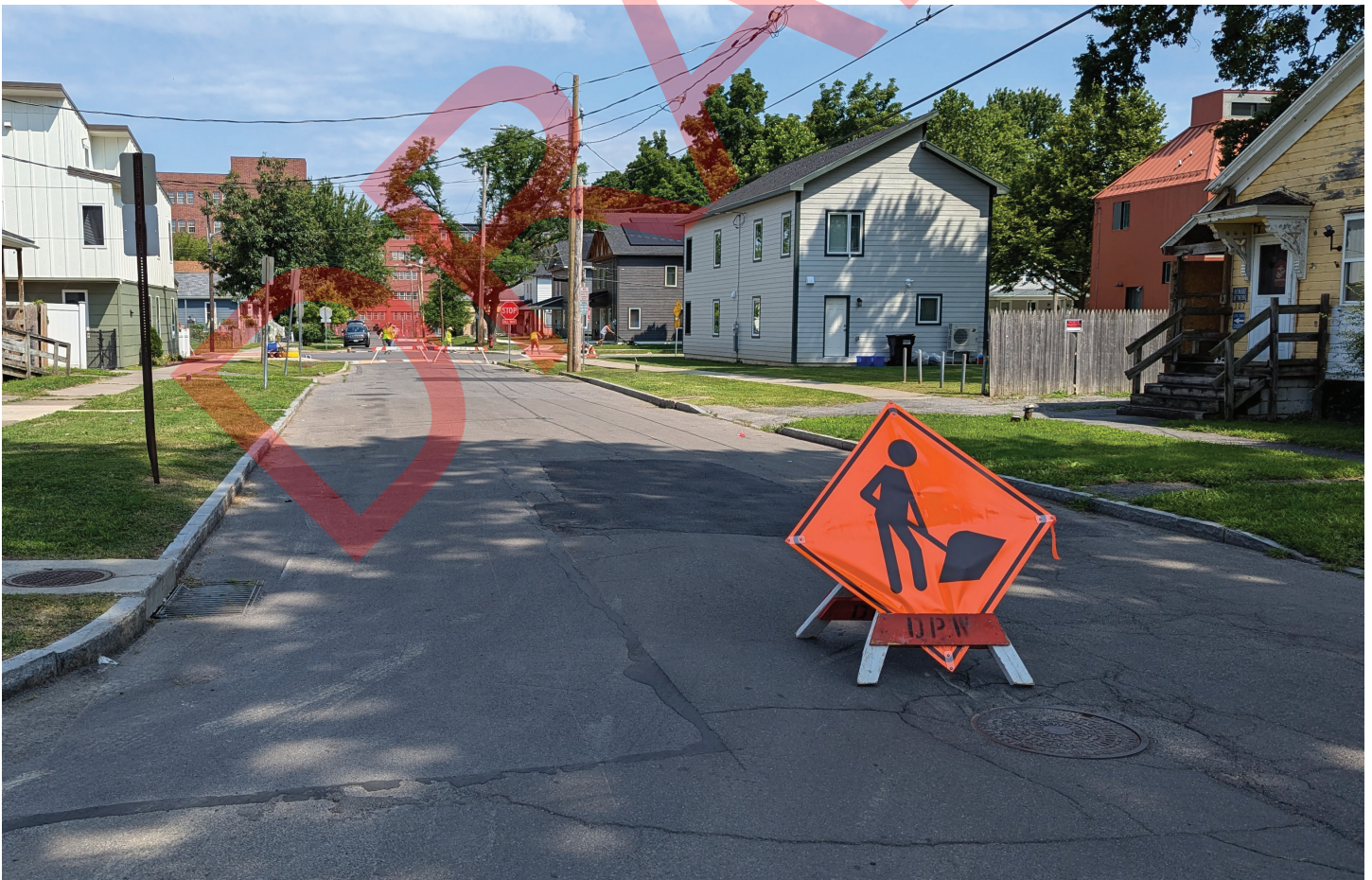
Temporary traffic control signs utilized during the installation of the Alchemical Nursery project.
