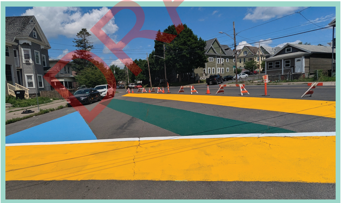
Large painted stripes were intended as a transition zone between vehicle traffic and the temporary pedestrian plaza on the Northside.
