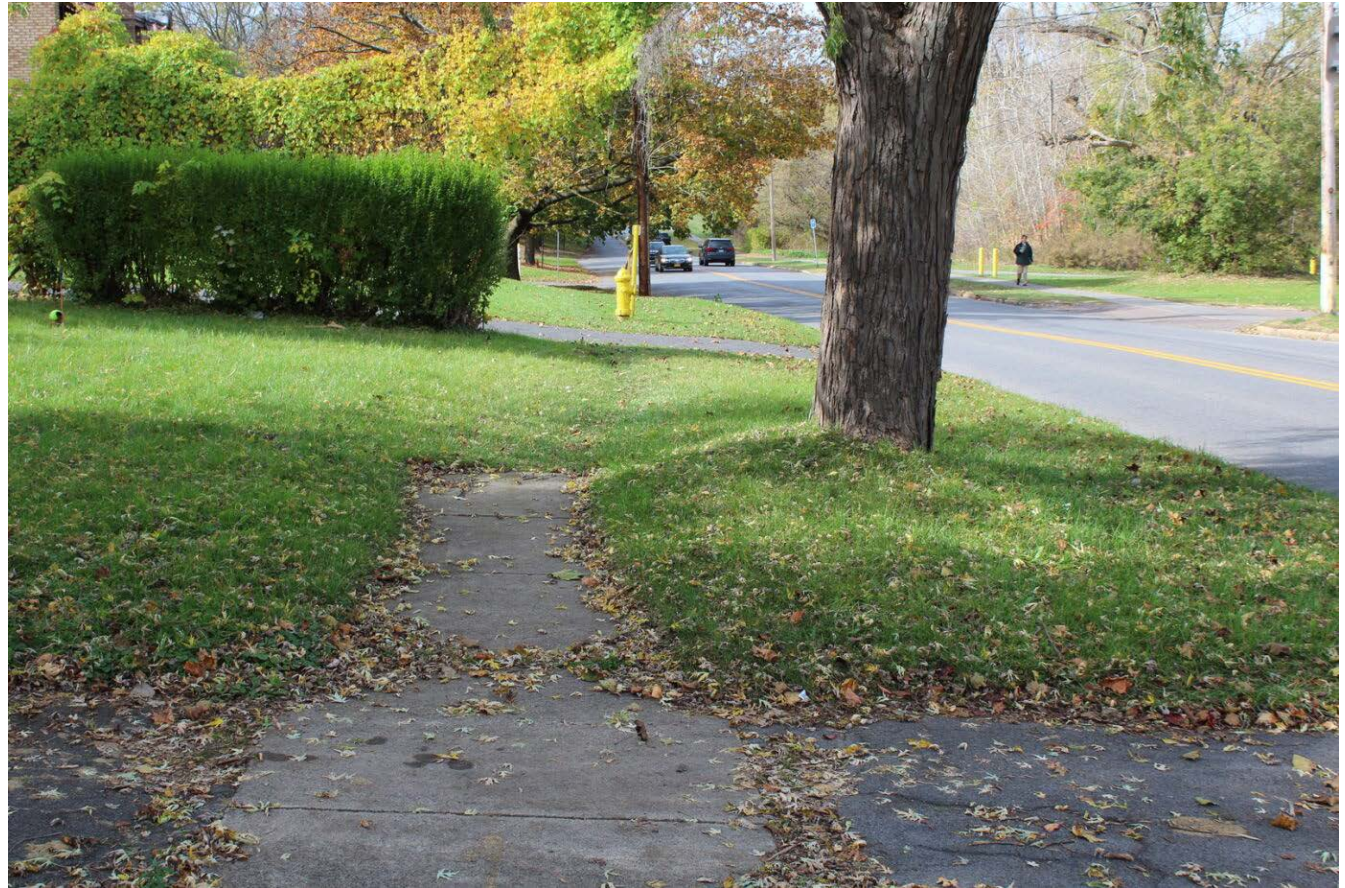
Missing Sidewalk on W Onondaga St
