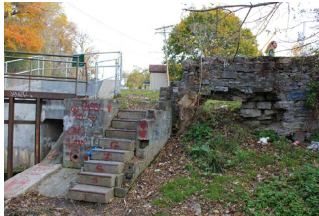
Stairs by Harbor Brook
