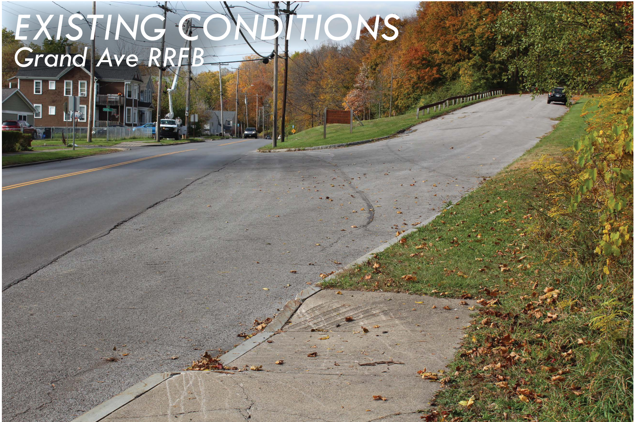
Figure 38a: Existing Conditions - Grand Ave RRFB
