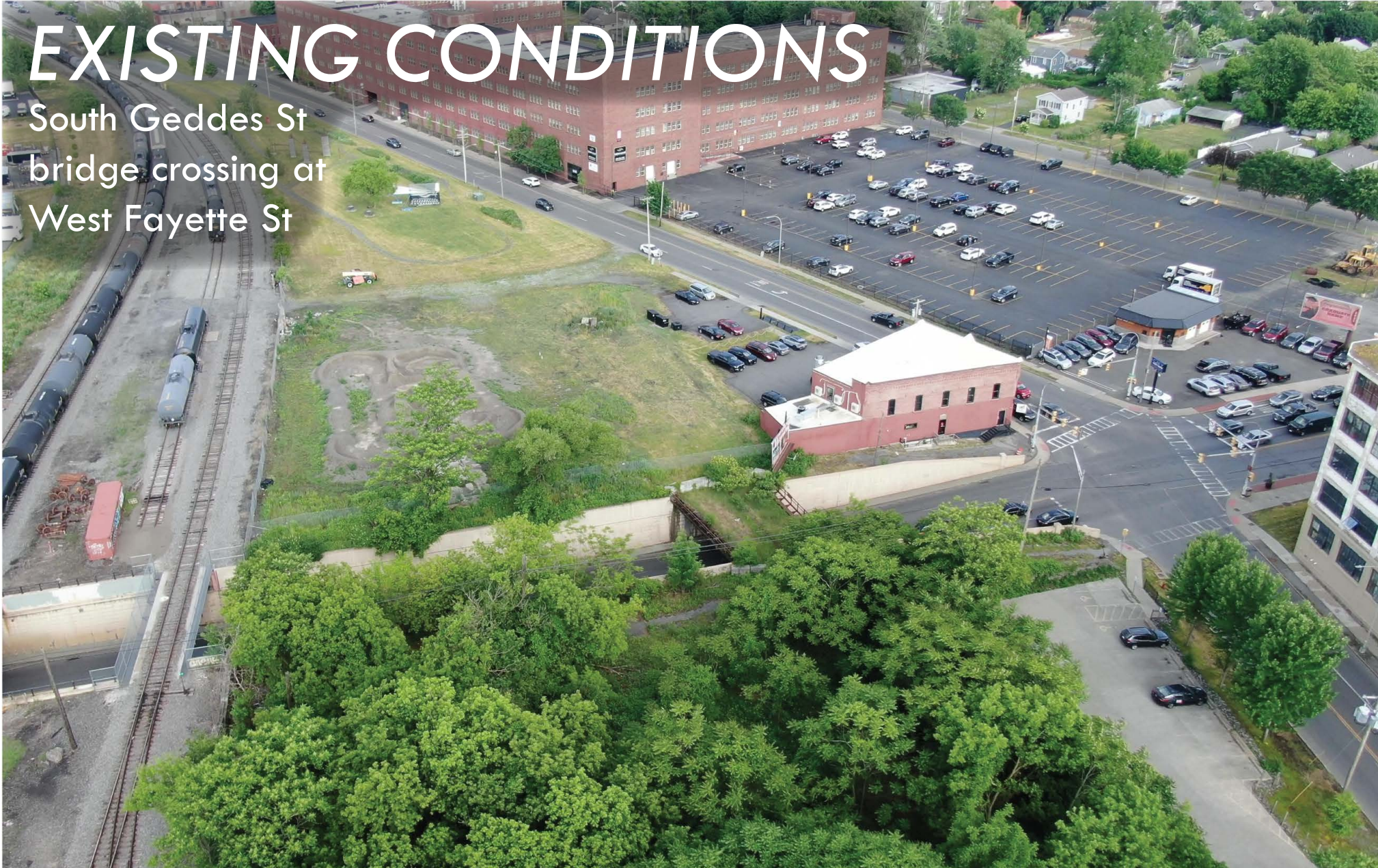
Figure 45a: Existing Conditions - S Geddes St bridge crossing at W Fayette St
