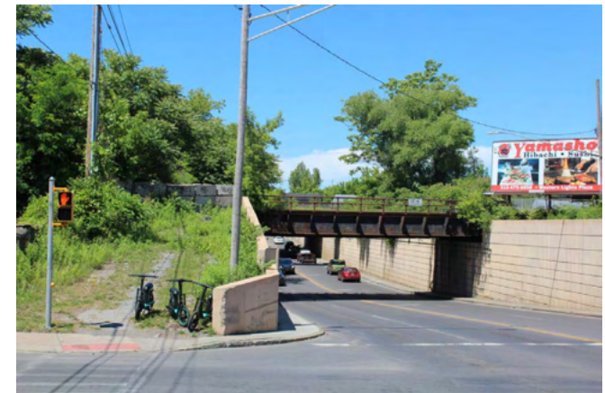
Abandoned Railroad Bridge over Geddes St
