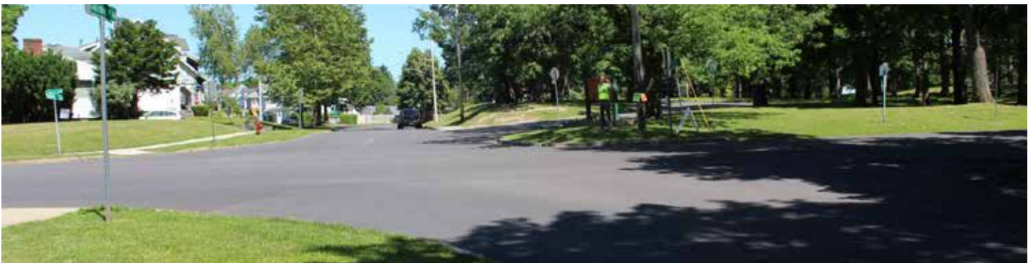
Salisbury Rd intersecting with S Avery Ave at Burnet Park - looking east
