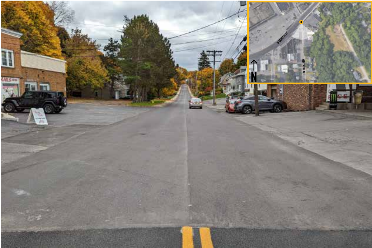
Figure 6.17: Existing conditions, Montrose Ave - looking south
