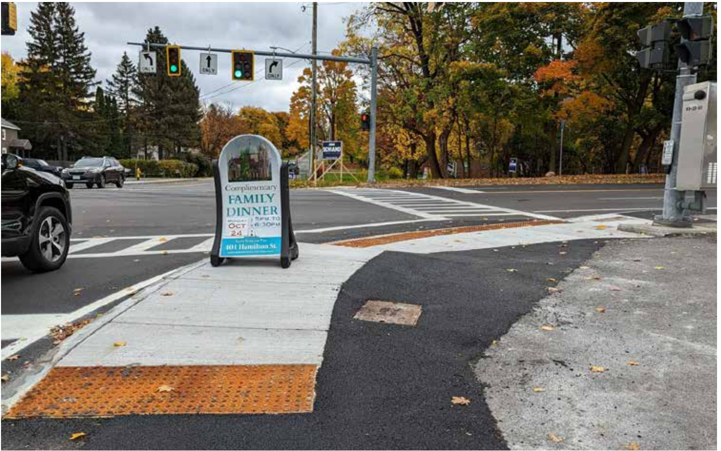
Pedestrian infrastructure on the northwest corner of W Genesee St & Fay Rd
