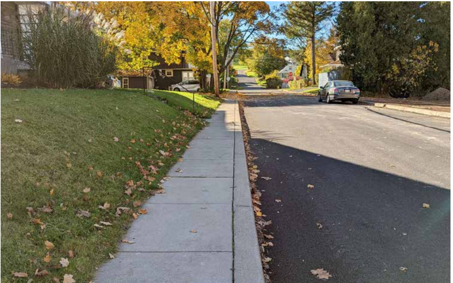
Sidewalk along the southern side of Rosita St
