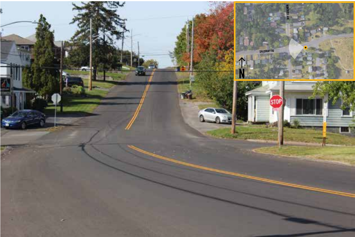
Figure 6.21: Existing conditions, Salisbury Rd - looking west
