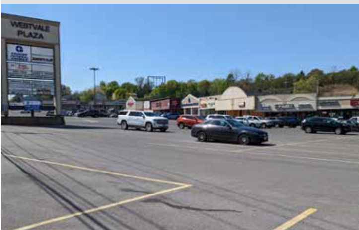
Parking lot at Westvale Plaza
