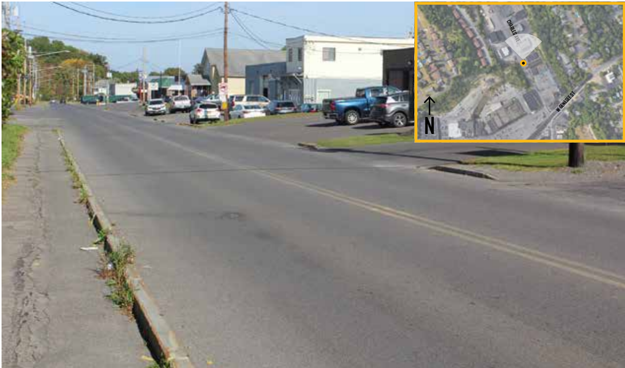
Figure 6.12: Existing conditions, Charles Ave - looking north
