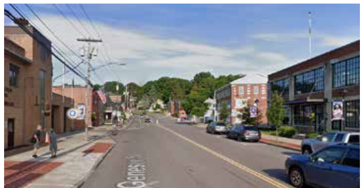
W Genesee St in Downtown Syracuse, Westvale, and the Village of Camillus. Source: Google Streetview
