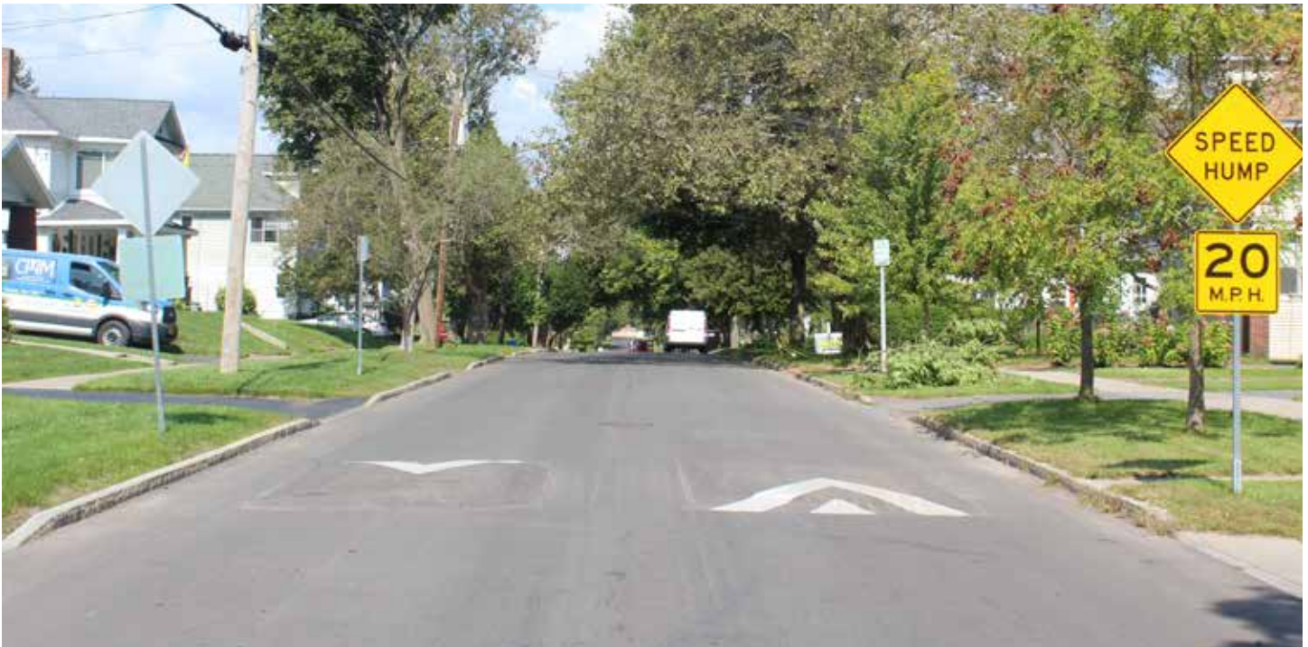
Speed cushions on Hickock Ave in Syracuse's Eastwood neighborhood
