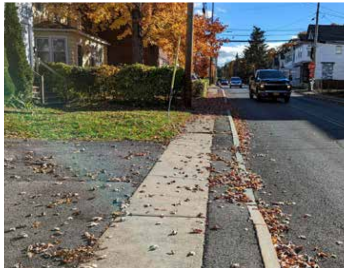
Narrow sidewalks on Charles Ave
