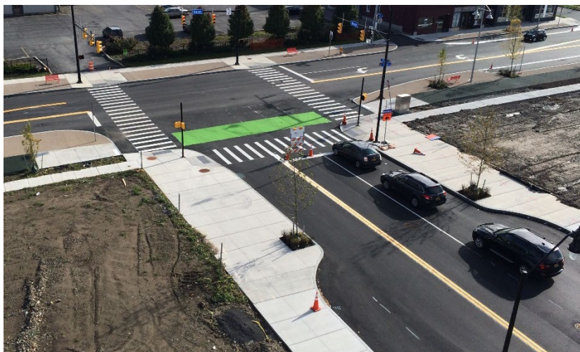
A view of the intersection of East Broad Street and Union Street after construction. (Source: Stantec)
