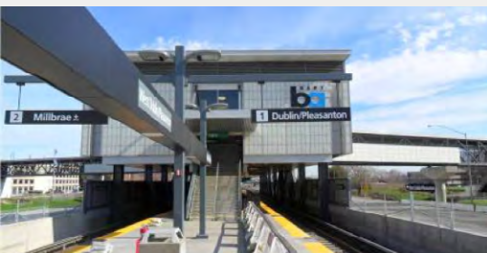
West Dublin/Pleasanton Station.
