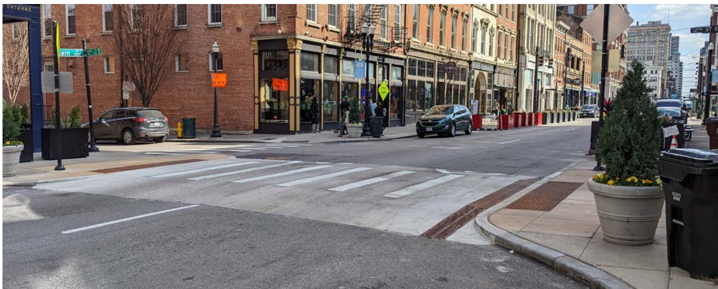
Speed management techniques from top: Chicane in Berkley, CA (Photo: NACTO); Speed cushion in Cincinatti, OH (Photo: City of Cincinatti); Raised crosswalk in Cincinatti, OH.
