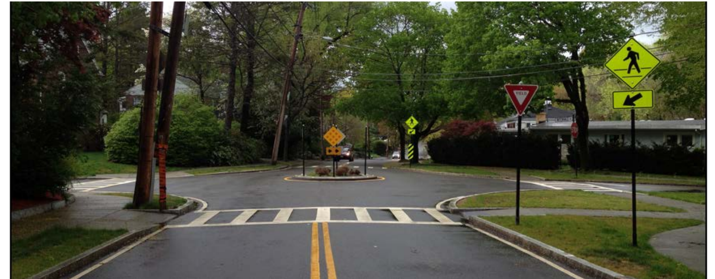
Mini-roundabouts, or traffic circles, slow vehicles down as they approach intersections while maintaining the flow of traffic. (Photo: NACTO)
