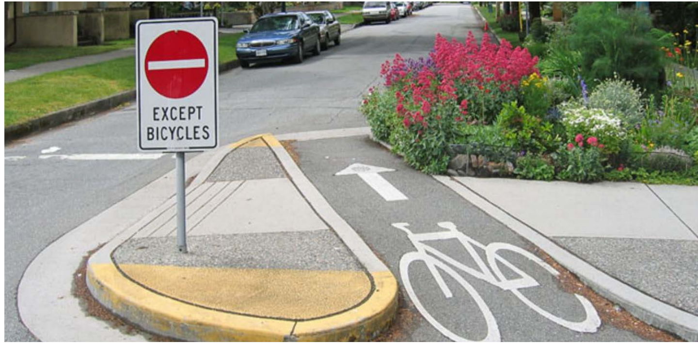
A diverter allows bicycles to continue along a street while diverting traffic. (Photo: NACTO)
