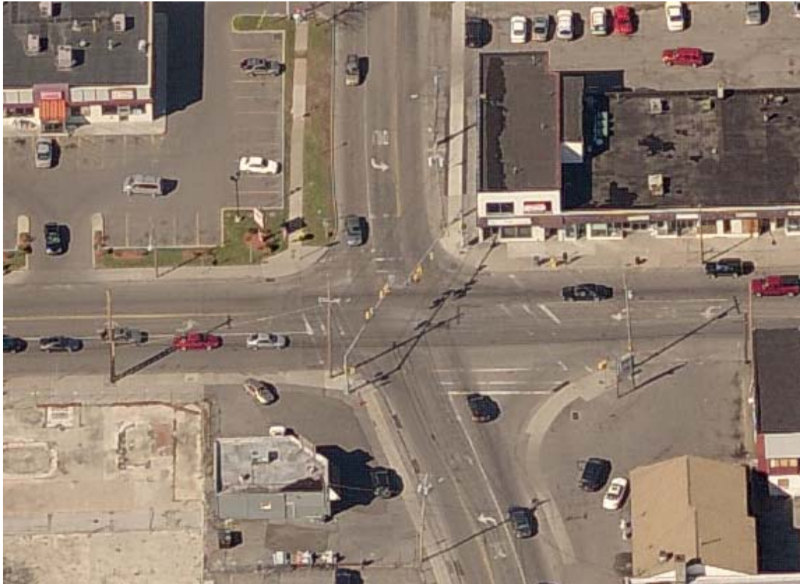
Aerial photo of James Street – S. Midler Avenue intersection (looking north)
