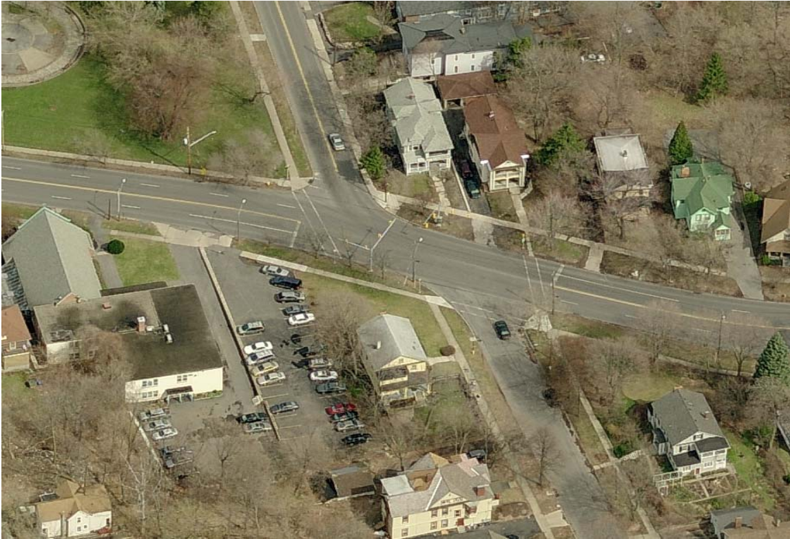
Aerial photo of East Genesee Street – Columbus Avenue intersection (looking north)
