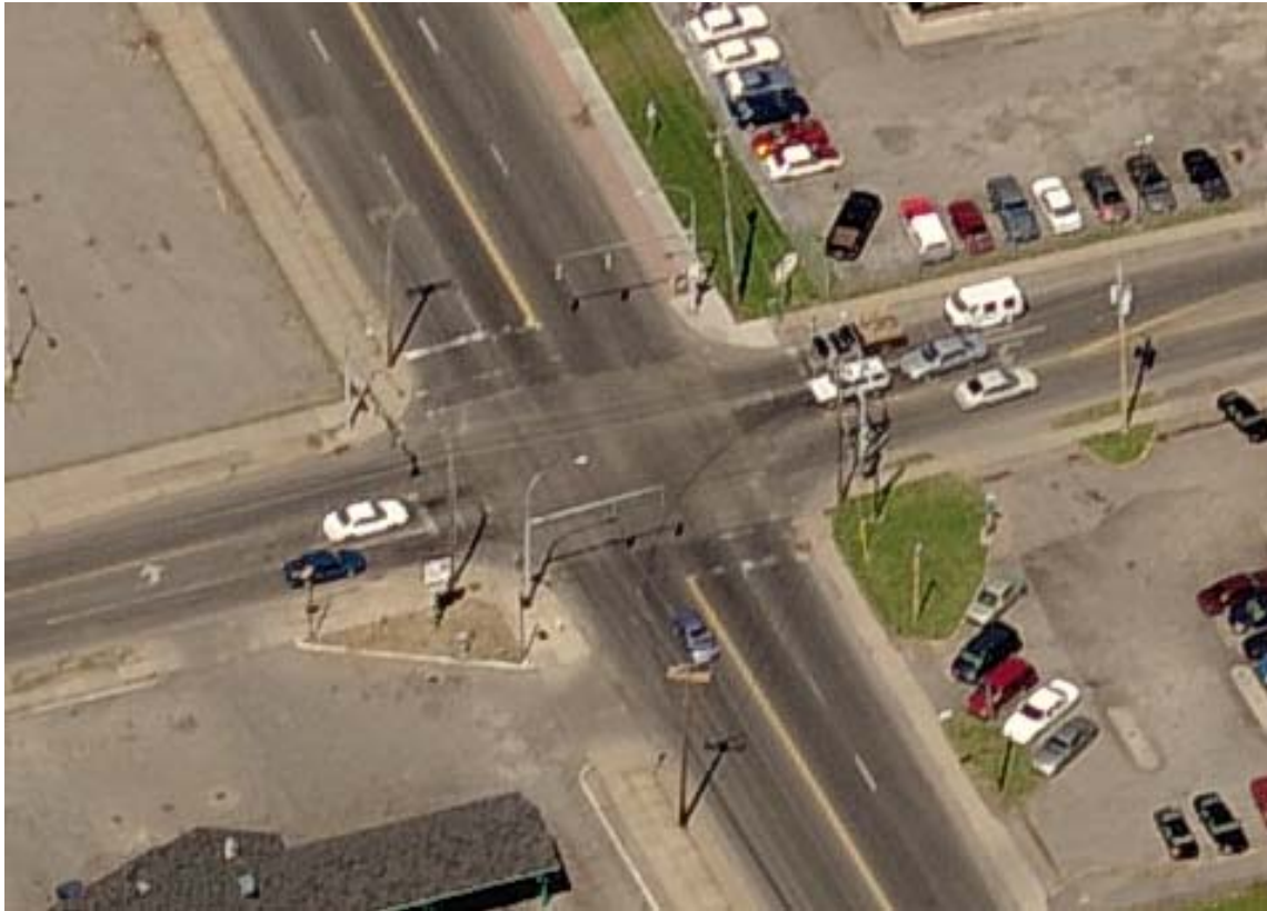
Aerial photo of S. Salina Street–Castle Street intersection (looking north)
