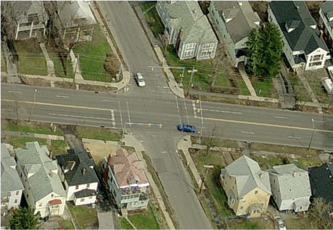
Aerial photo of East Genesee Street – Westmoreland Avenue intersection (looking north)
