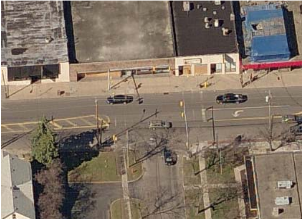
Aerial photo of James Street – Hickok Avenue intersection (looking north)
