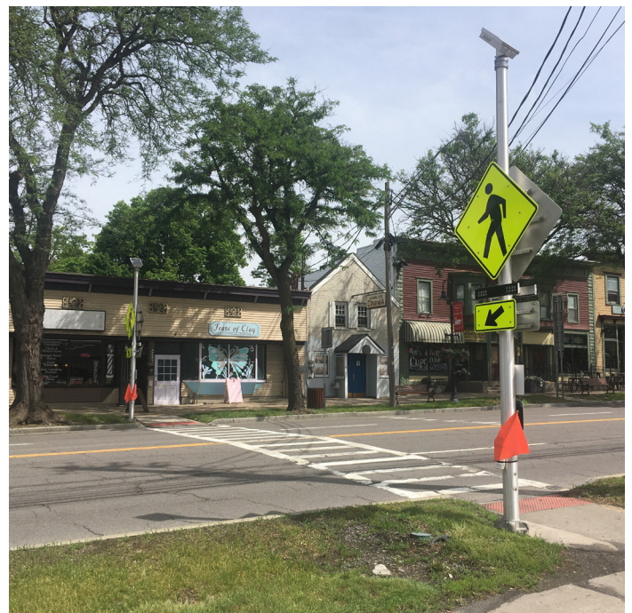
The existing mid-block crosswalk on Route 173 utilizes rectangular rapid flashing beacons (RRFBs) to alert drivers.
