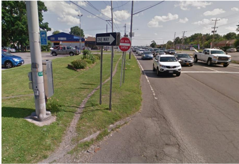
Image 3 - Signed bus stop location with ADA accessibility sign at the southeast corner of US 11 / Sand Road. Image is taken looking south. A worn footpath is visible. No sidewalks, curb cuts, or other accessible amenities are provided.
