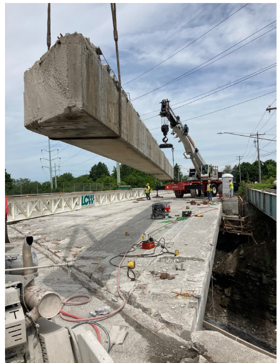
E Brighton Ave Bridge over railroad. Source: Syracuse
