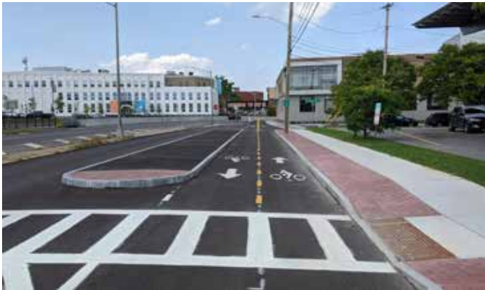
Figure 4-17. Separated bike lanes are exclusive facilities for bicyclists that are distinct from the sidewalk and physically separated from motor vehicle traffic with a vertical element.
