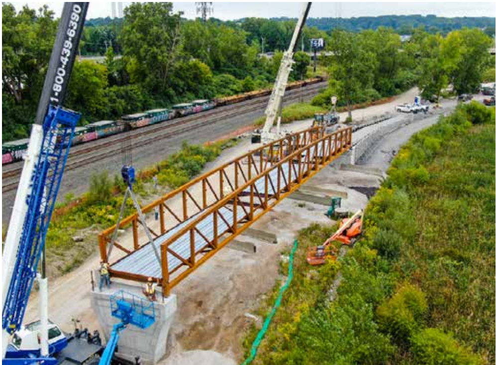
Construction of a new Onondaga County Loop the Lake Trail bridge.
