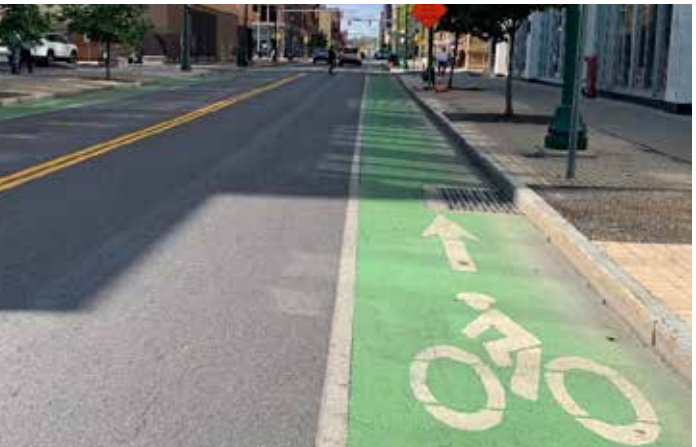
Figure 3-7. Bike lanes establish an area for exclusive bicycle use outside the path of motor vehicles.
