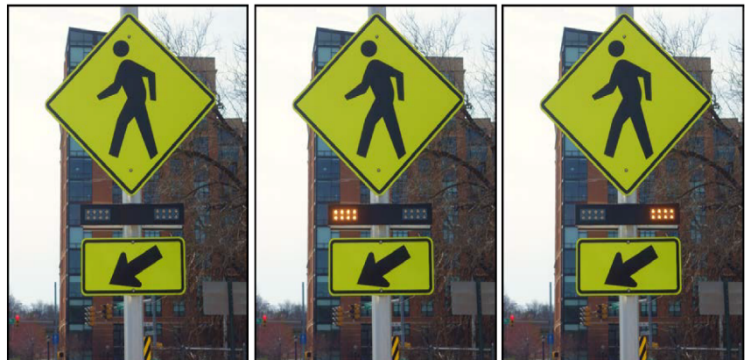
Example of an RRFB dark (left) and illuminated during the flash period (center and right) mounted with W11-2 sign and W16-7P plaque at an uncontrolled crosswalk. Source: FHWA Interim Approval for Optional Use of Pedestrian-Actuated Rectangular Rapid-Flashing Beacons at Uncontrolled Marked Crosswalks, 2018.
