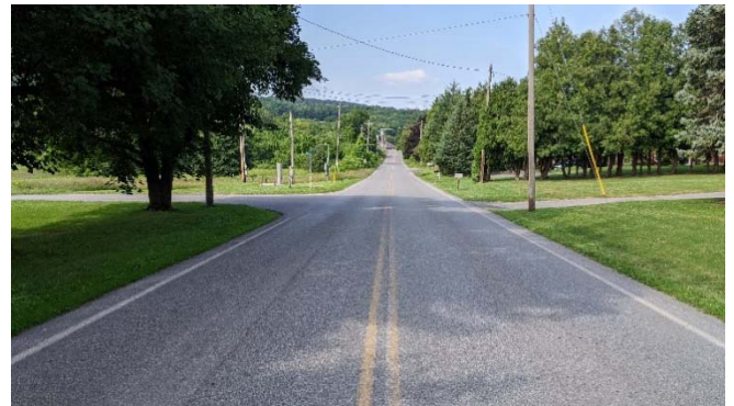
Tuscarora Road near Tom Tom Street facing west
