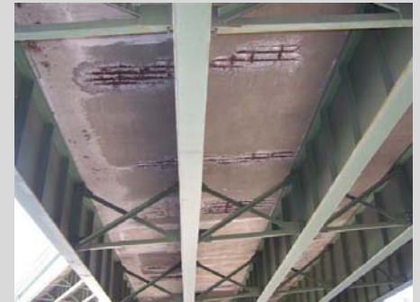
Deterioration on the underside of a bridge.
