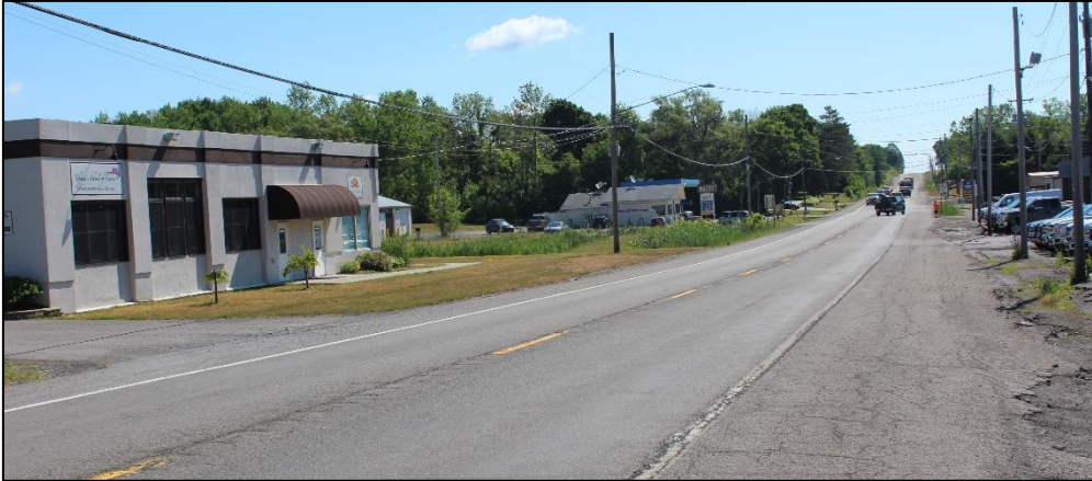
Existing conditions in the study area's Highway Commercial district
