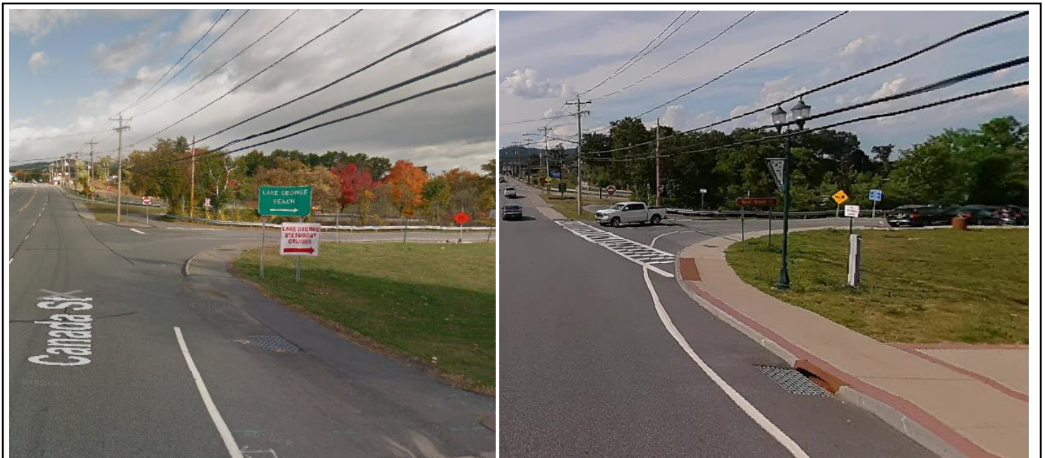
Figure 7: The U.S. 9 gateway to Lake George before (left) and after (right) streetscape improvements. (Imagery from Google Street View)
