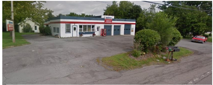
The existing structure and streetscape at 1321 U.S. 20
