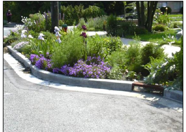
Curb cuts can be designed to direct stormwater runoff into vegetated areas
