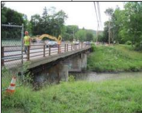
Seneca Turnpike over Onondaga Creek City Syracuse
