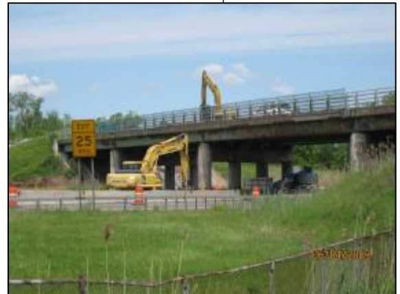
Bartel Road over Interstate 81, Cicero Recipient of 2009 ARRA funding
