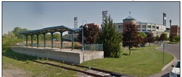
Image 10 – Abandoned OnTrack Passenger Platform near NBT Bank Stadium behind the Regional Market
