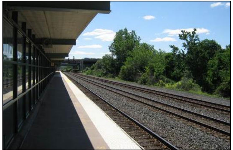
Image 8 – Amtrak Passenger Platform, RTC, Syracuse, NY
