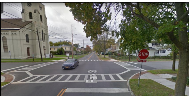
Image 11 – Park Street Greenway Improvements (Sharrows, Ladder Crosswalks, Curb Ramps) – Park Street at Turtle Street.
