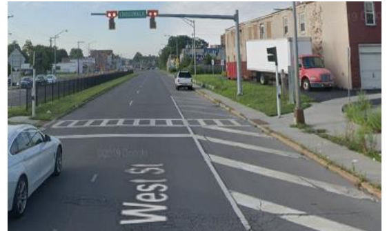
West Street crosswalk at end of Otisco Street (image courtesy of Google Maps).
