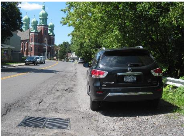
Informal parking lane, West Fayette. Street.
