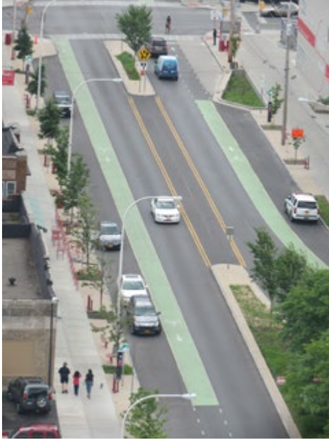
Green bike lanes, green medians, street furniture, and new sidewalks along East Genesee Street were installed as part of Phase I of the Connective Corridor in late fall 2012.
