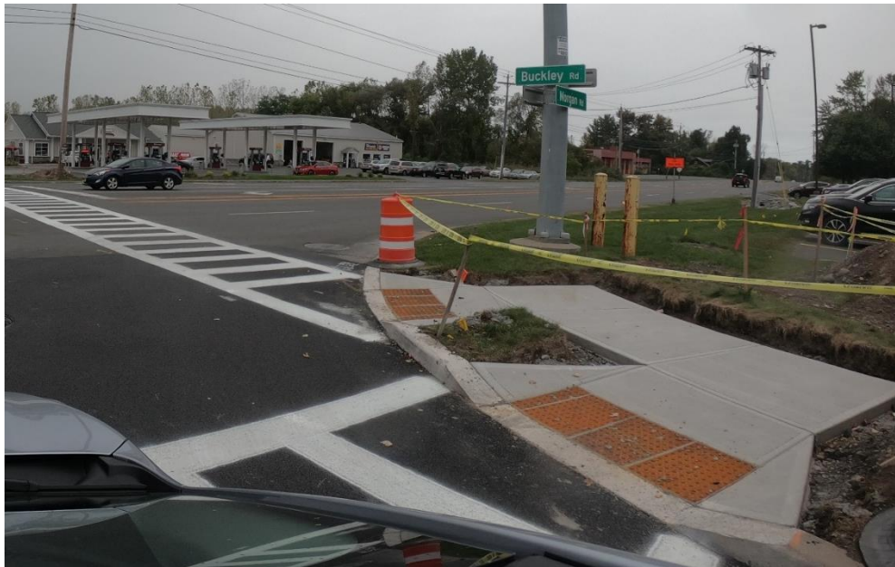
Image 1 – Morgan Road/Buckley Road Intersection – repaving, restriping, and pedestrian facilities under construction.
