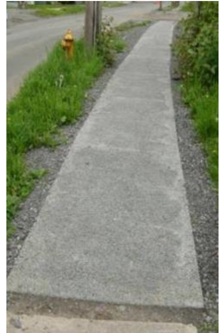
Figure D-2: Grand Avenue Porous Pavement Sidewalk Test Segment
