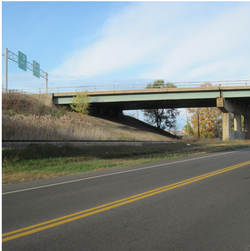
Milton Avenue under NYS 5 Bridge in Camillus
