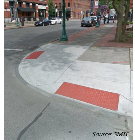
Figure 18: Truncated domes. ADA-compliant truncated domes at the intersection of Franklin and Jefferson Streets
