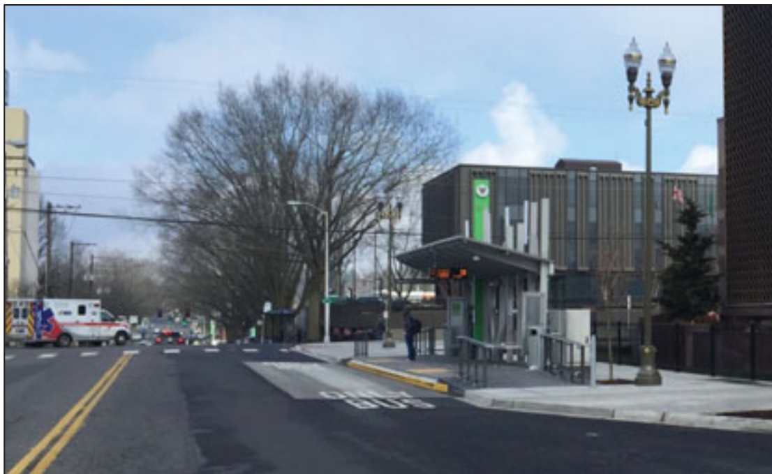
Figure 39: C-TRAN "The Vine" BRT station in Vancouver, WA showing mixed-traffic configuration with targeted infrastructure improvements including station, sidewalk, bus pad, and pavement/ADA ramp improvements. (Source: IBI Group)
