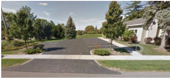
Example of concrete sidewalk extending over driveway
