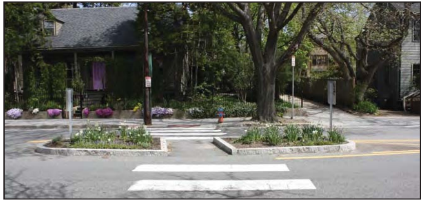
A raised median with vegetation could be added at the Velasko Road/Western Lights Plaza driveway intersection, given a minor road widening.
