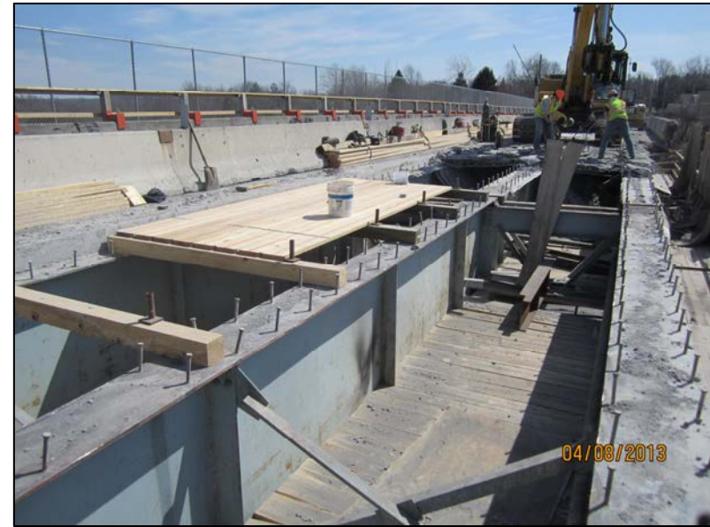
Fremont Road over CSX rail road Bridge deck replacement
