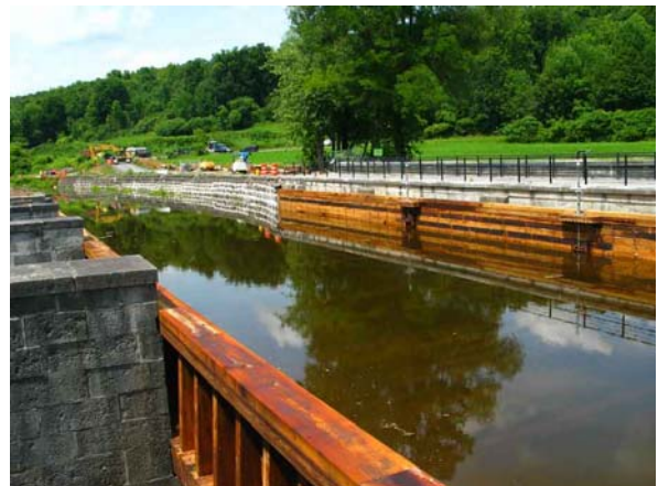
Camillus Erie Canal Park - Nine Mile Creek Aqueduct Restoration Project ( www.eriecanalcamillus.com/aqueduct.htm )
