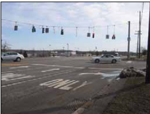
A lack of shoulders on Route 31 near the Route 481 interchange makes this area challenging for cyclists. (Top: Looking west along Route 31 at the Route 481 interchange. Bottom: Looking east along Route 31 near the Marketfair North entrance).
