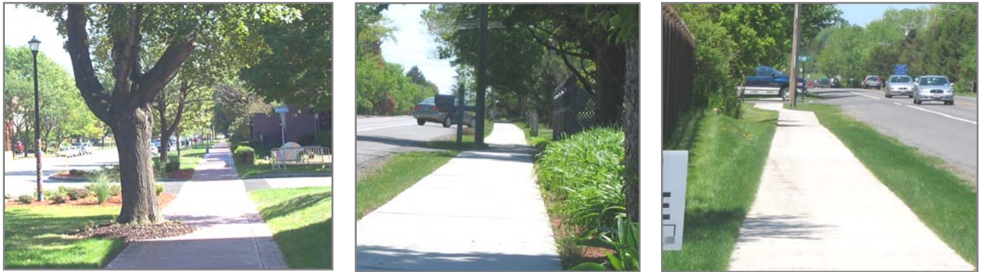
Sidewalk built around a mature tree on University Ave. in Rochester, NY (left); Sidewalk “cut-out” to accommodate utility pole on Route 92 in Village of Manlius, NY (middle); Sidewalk meandered to avoid utility pole on Route 92 in Village of Manlius, NY (right).
