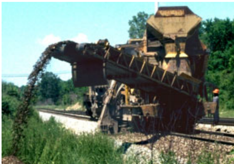
CSXT Track Maintenance Crew undercutting rail and cleaning ballast.
