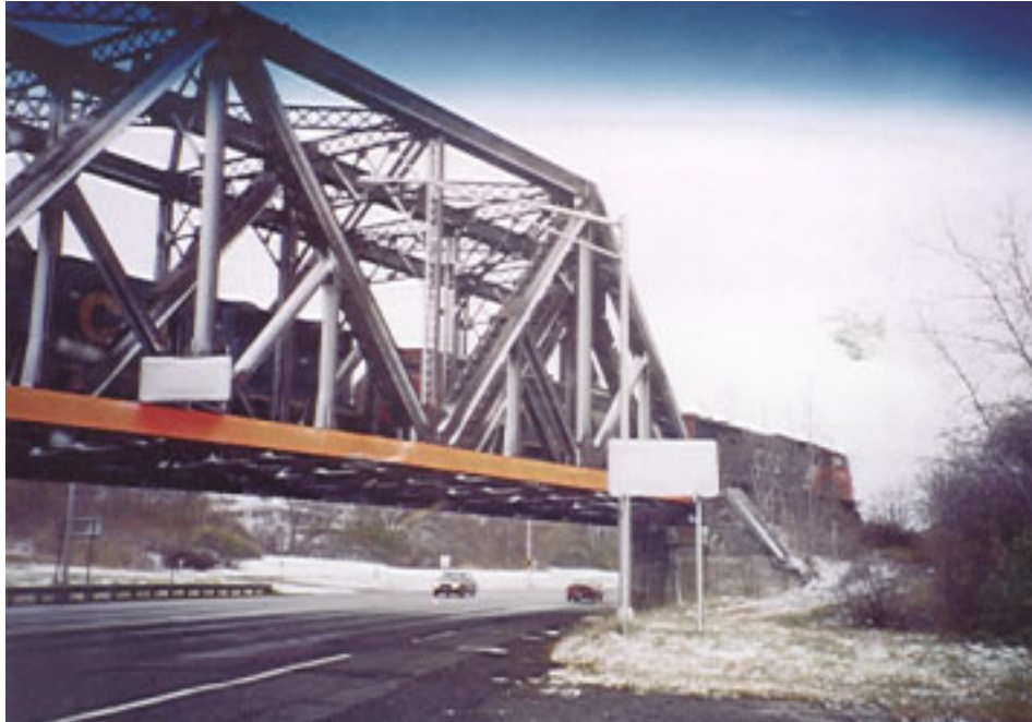
Southbound Canadian National/CSXT Freight Train over Onondaga Lake Parkway
