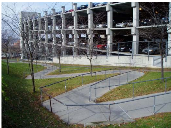
The access from this parking deck across from the Carrier Dome illustrates the challenges of ADA compliance on University Hill's steep grades.
